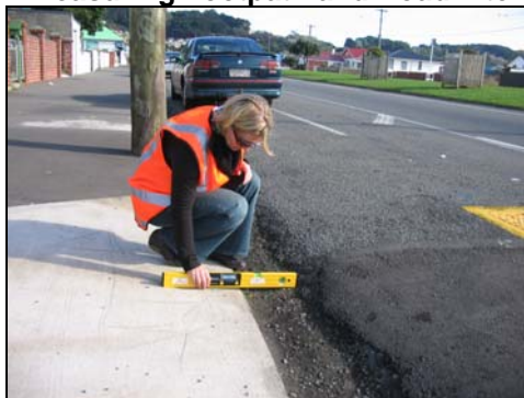
Measuring footpath gradient
