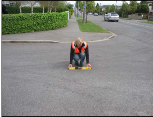
Figure RC31.1 Measuring Road Crossing Cross Fall
