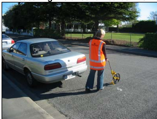
Figure PL42.1 Measuring Distance to Nearest Traffic Lane
