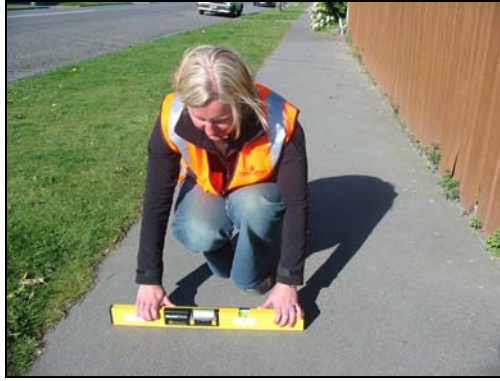
Figure PL36.1 Example of Measuring Cross Fall
