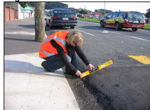
Measuring road gradient
