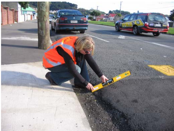
Figure 4.3 Road Crossing – Possible Tripping Hazard
