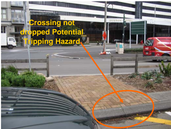
Figure 4.2 Vehicle Parking Intruding onto Road Crossing & Possible Tripping Hazard
